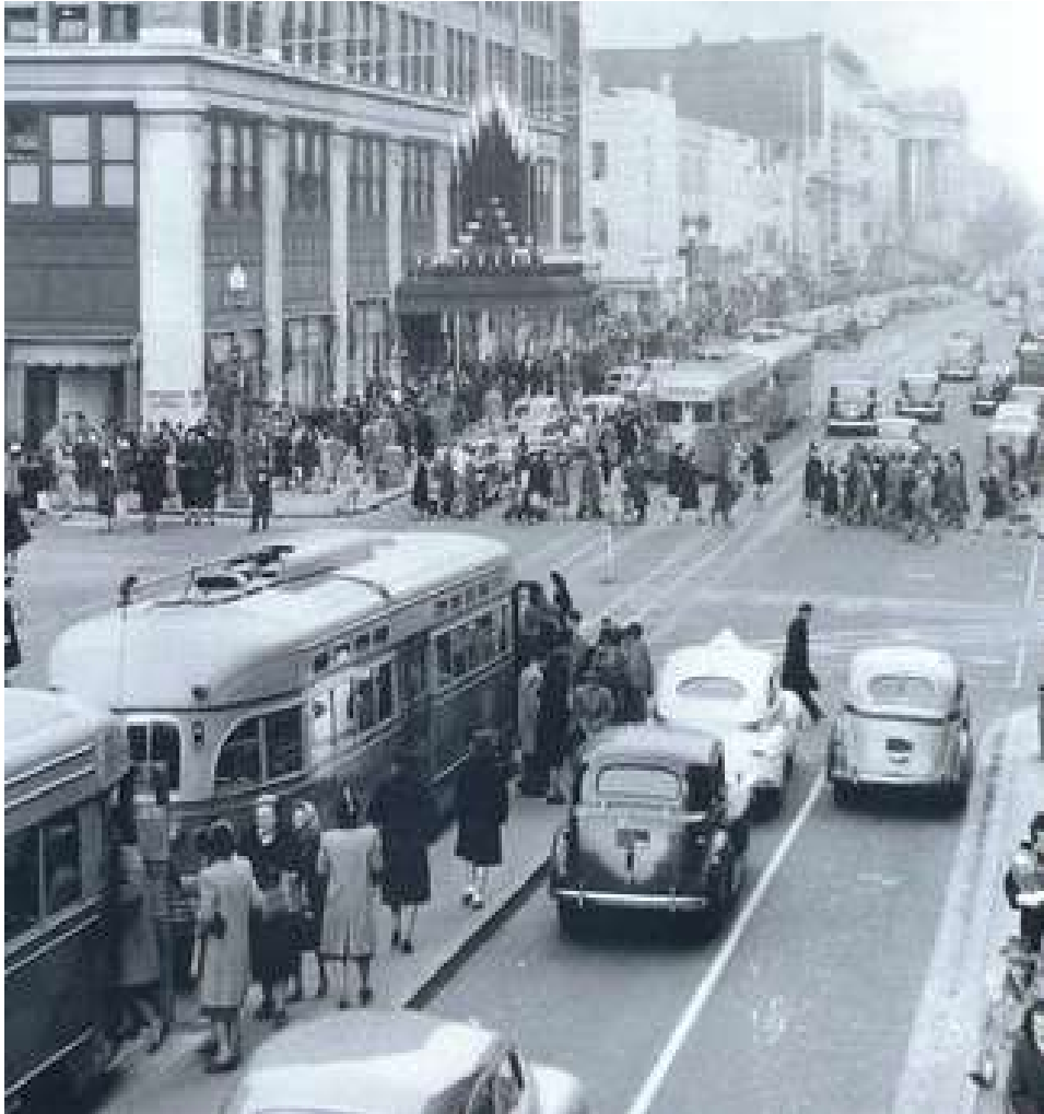
(Washington, DC View East Down F Street NW)
